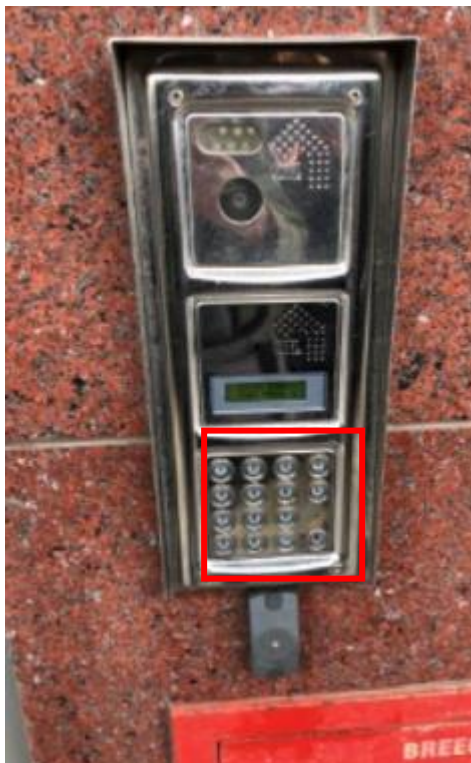
Figure 2-8 Core 4 Test Apartment block buzzer/ intercom
