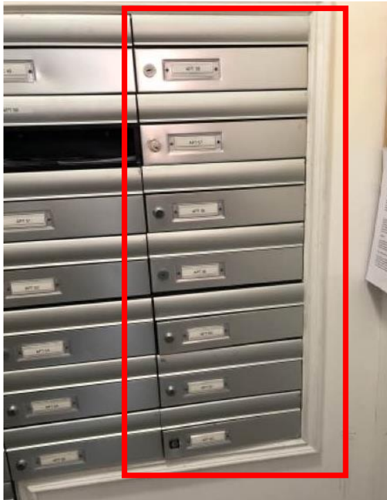
Figure 2-3 Core 4 Test Apartment block post boxes (RHS)
