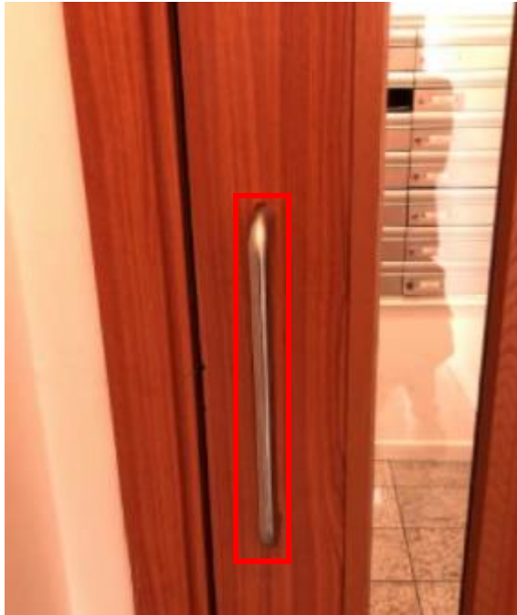
Figure 2-7 Core 4 Test Apartment block Lobby interior door handle
